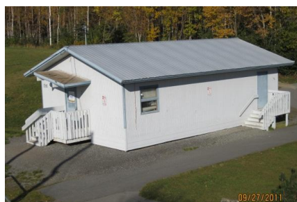
Figure 1: View of Chinook Elementary Relocatable Classroom
