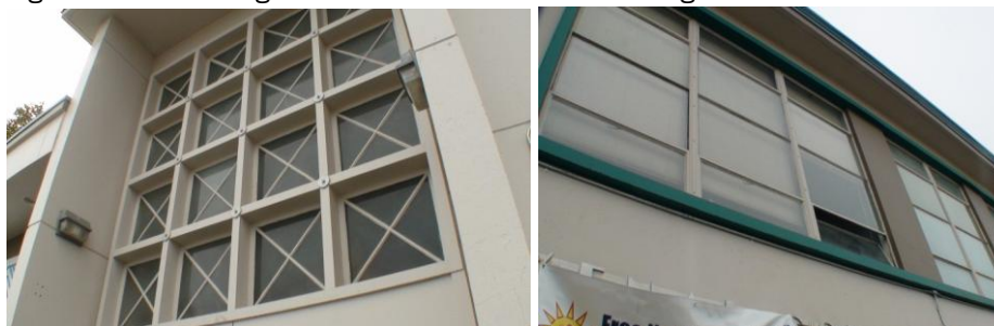
Figure 2: View of Single Pane Windows and North Facing Windows
