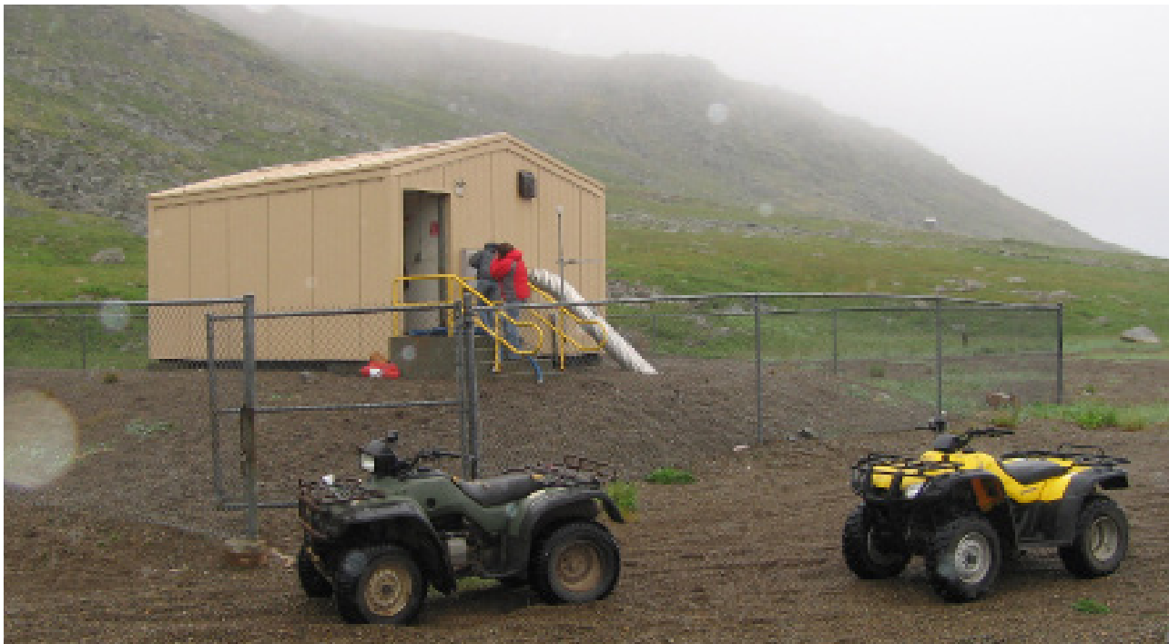
Workers enter the water well plant in Gambell. Photo: Department of Commerce, Community and Economic Development; Division of Community and Regional Affairs' Community Photo Library.
