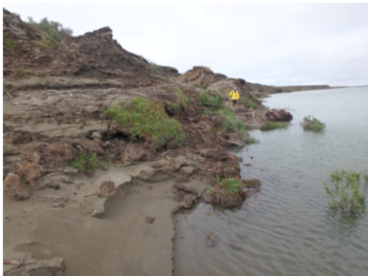
Sand, soil, and vegetation on this beach are being eaten away by coastal erosion. Photo credit: Matthew Whitley
