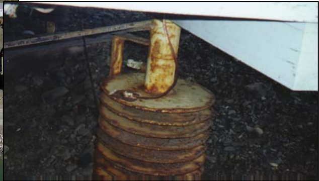
Library pilings in 2000
